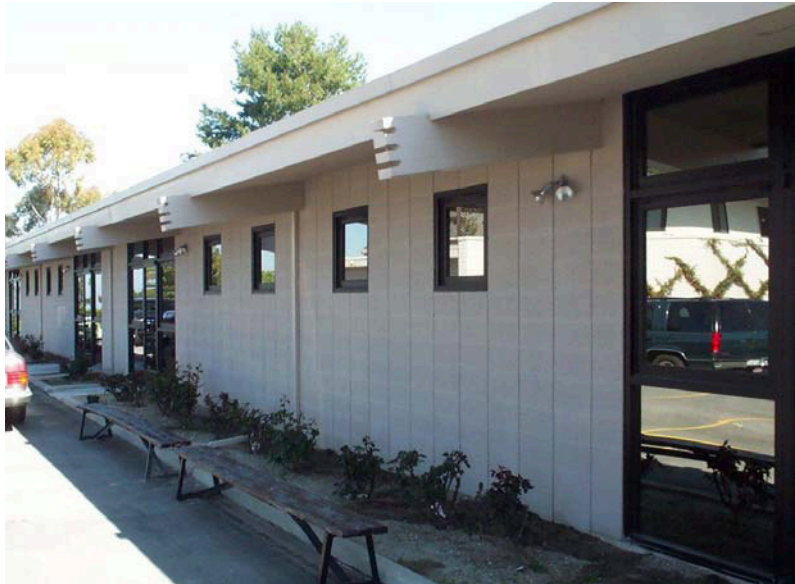
Figure 3. Overhanging eaves will help greatly to prevent moisture from entering this stack bond CMU wall.
