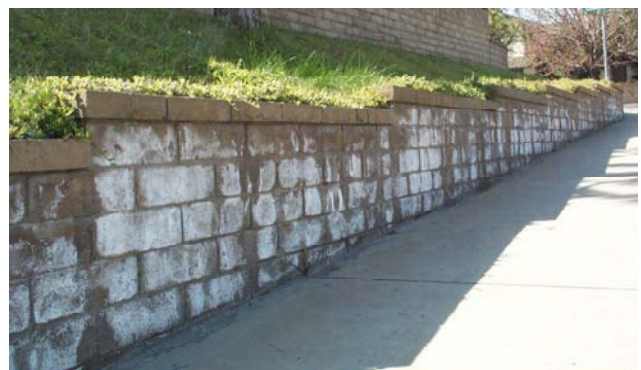
Figure 1. Typical white efflorescent salts on brick and block masonry
