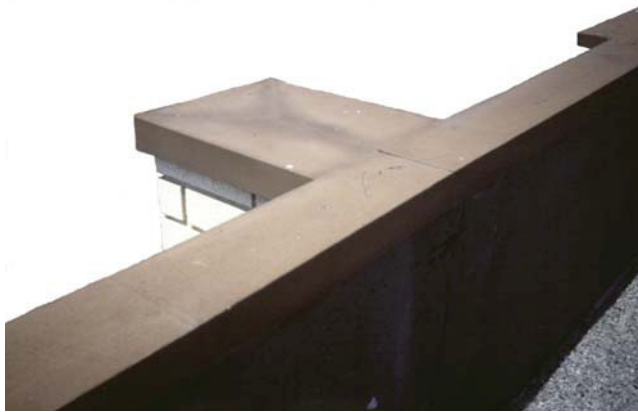
Figure 4. A full metal coping helps in waterproofing a wall and eliminates moisture penetration through the tops of parapets
